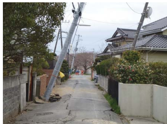
Photo 1 Liquefaction damage due to the 2011 off the Pacific coast of Tohoku Earthquake in Sawara city. (photo by Kentaro Nakai on April 3, 2011.)
